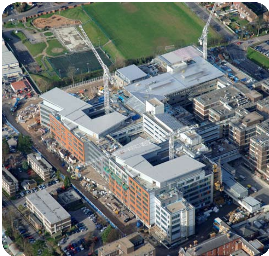
Queen Alexandra Hospital, Portsmouth
